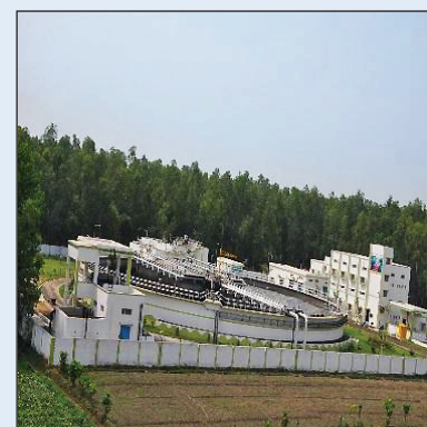
Treatment Plant, Haridwar
