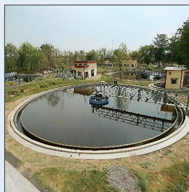
Treatment Plant, Allahabad
