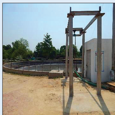
Treatment Plant, Kanpur
